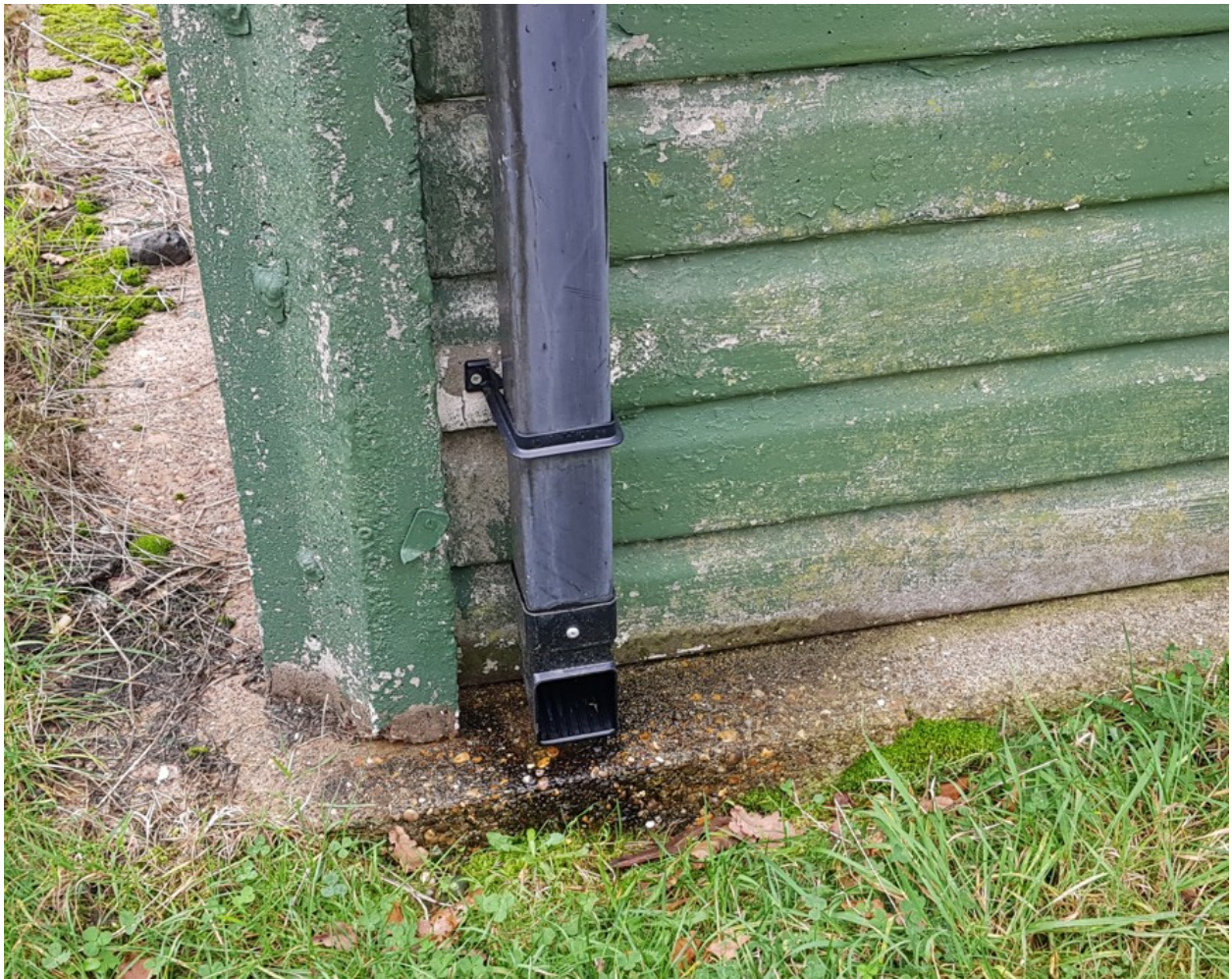
Figure 3: Existing Drainage arrangement
